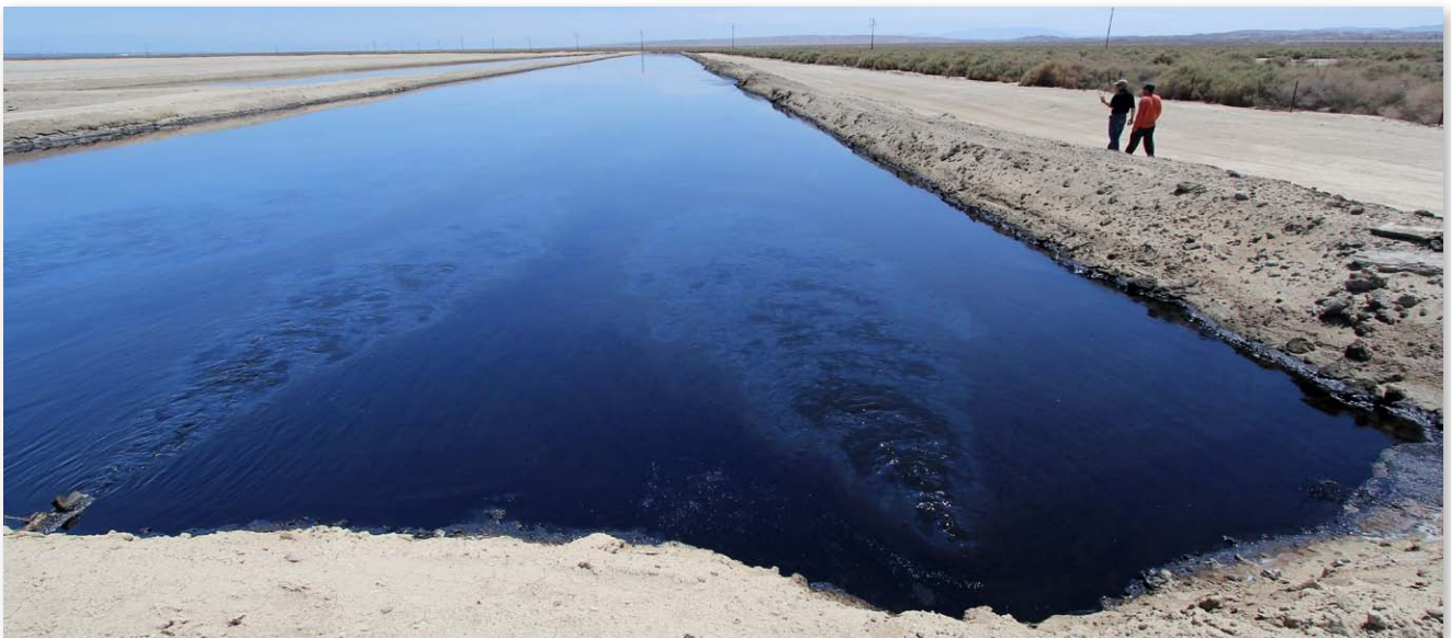
Image A: Unlined wastewater disposal pit in Kern County, CA.
